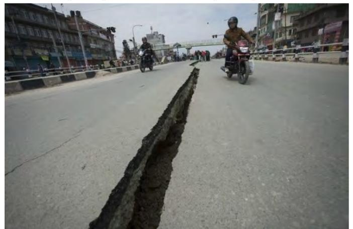
A crack in a road near Kathmandu caused by the earthquake.
